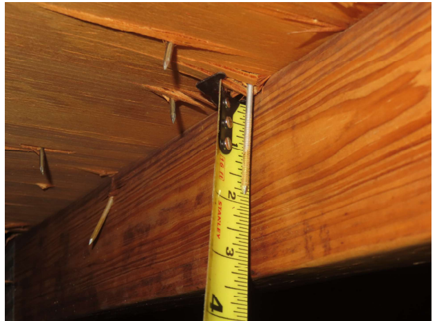
Roof deck attachment - 8d nails
