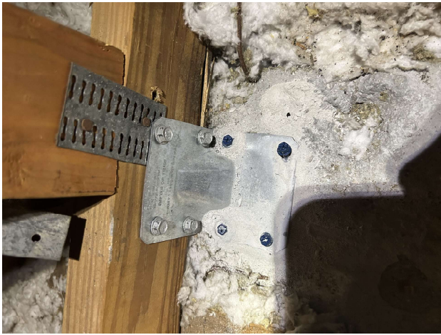
Roof to wall attachment - Clips
