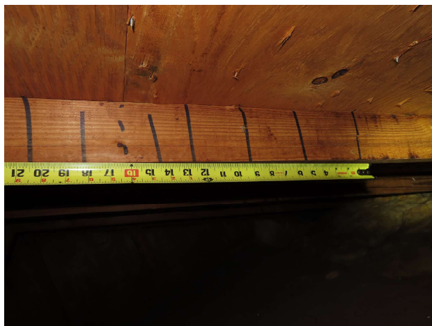
Roof deck nail spacing - Edge
