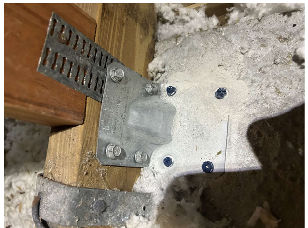
Roof to wall attachment - Clips
