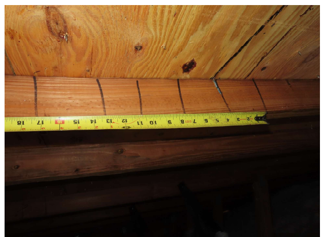
Roof deck nail spacing - Field
